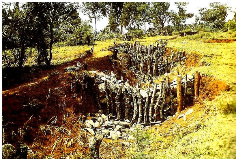
**Check dam to control gully erosion**
